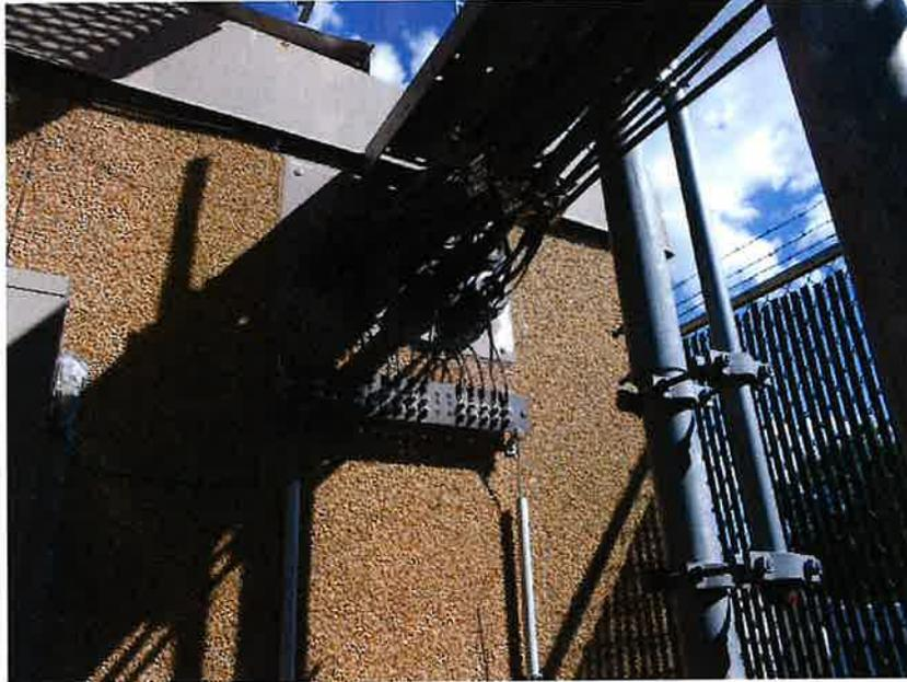
Photo of existing hatch plates and ground bar at shelter.
