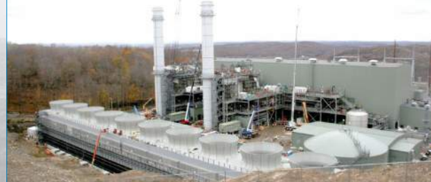
Kleen Energy Generating Facility
