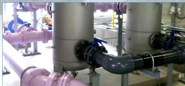
UConn Reclaimed Water Facility
